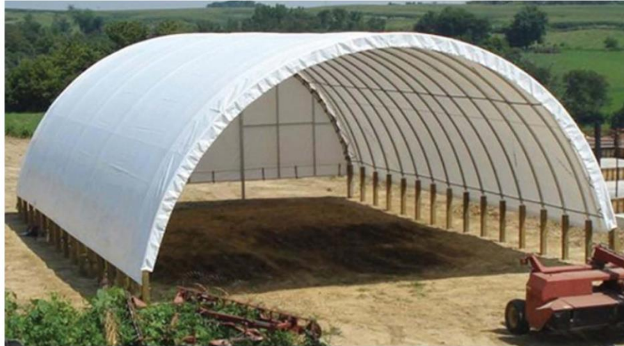
Actual image of a 38' x 40' arch building, wood post foundation shown
